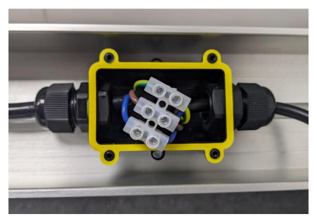
Ensure that the junction box lid is screwed down correctly and the gland is tightened to preserve IP rating.
